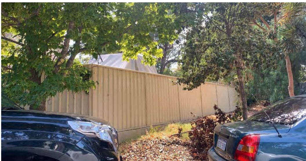
Fencing along the southern property boundary adjacent to the public open space and end of the cul-de-sac.
